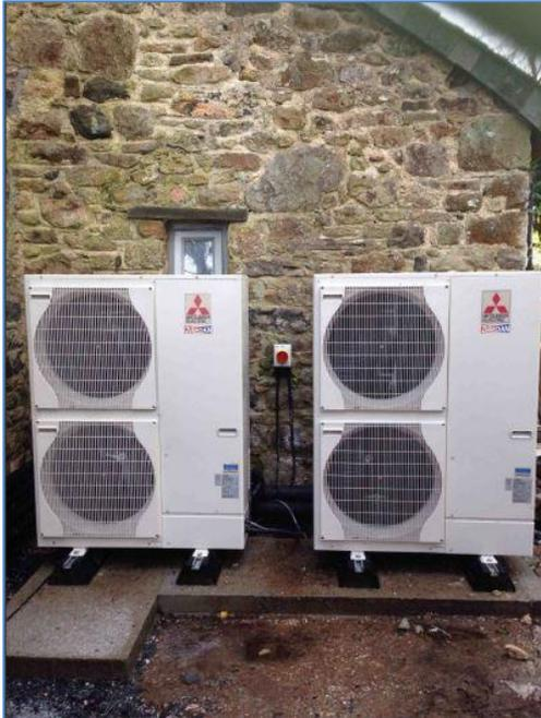
**ABOVE:** The two 14kW Ecodan units work together to meet the 20kW heat demand of the renovated farm buildings.
