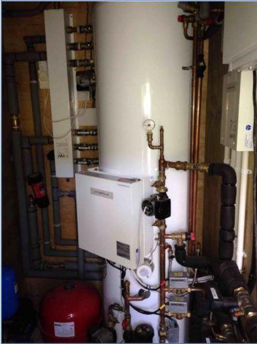
**ABOVE:** The 300 litre stainless steel hot water tank provides all the heating and hot water the newly renovated home needs.
