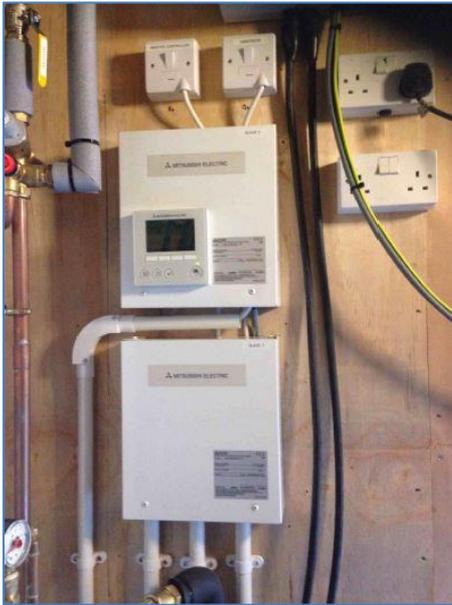
**ABOVE:** Ecodan's intelligent, self-learning controls decide which heating system to use at any time to ensure the house is heated in the most economical way possible.
