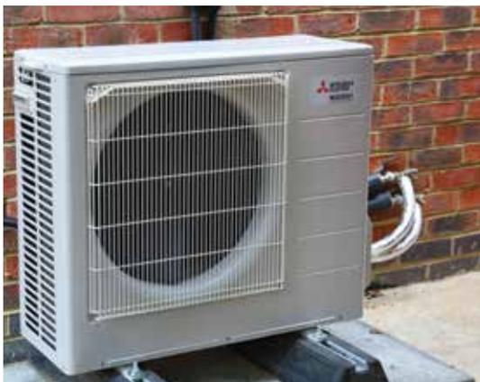
The Ecodan QUHZ outdoor unit sends renewable heat energy, harvested from the air to a thermal store, which then delivers hot water as required.
